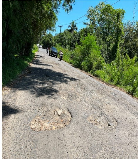
Figure 1. Pavement and Curve Conditions
