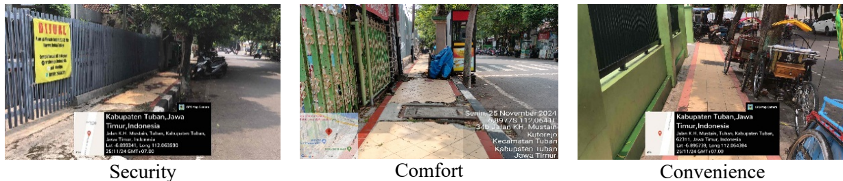
Figure 3. Condition of Pedestrian Path Segment 1
