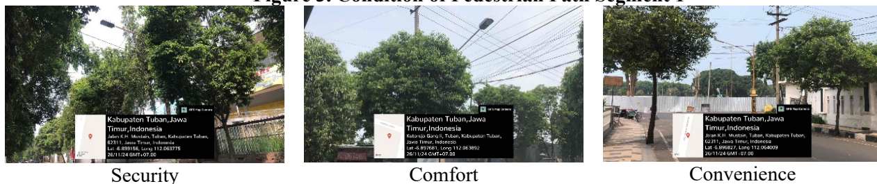
Figure 4. Condition of Pedestrian Path Segment 2
