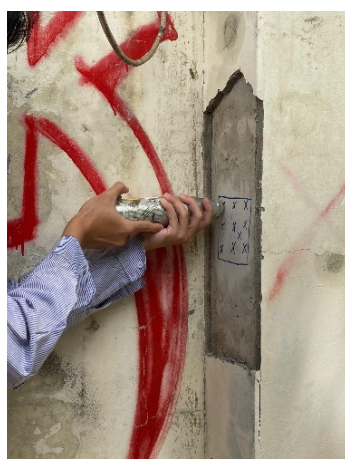
Figure 5. Schmidt Rebound Hammer Test
