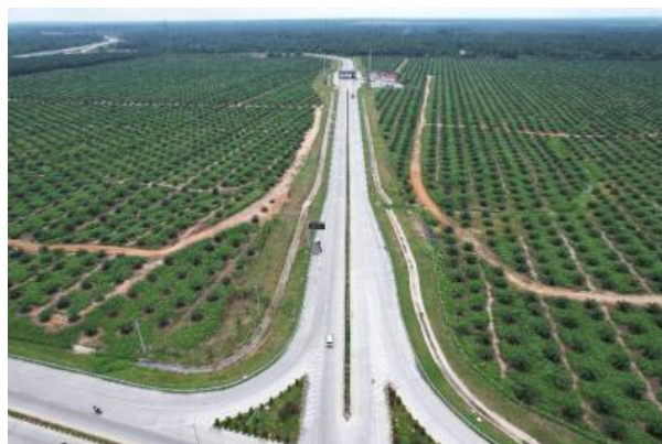
Figure 26 Trans Sumatra Toll Road Access Section – Lima Puluh Toll Gate Source: Author's Documentation
