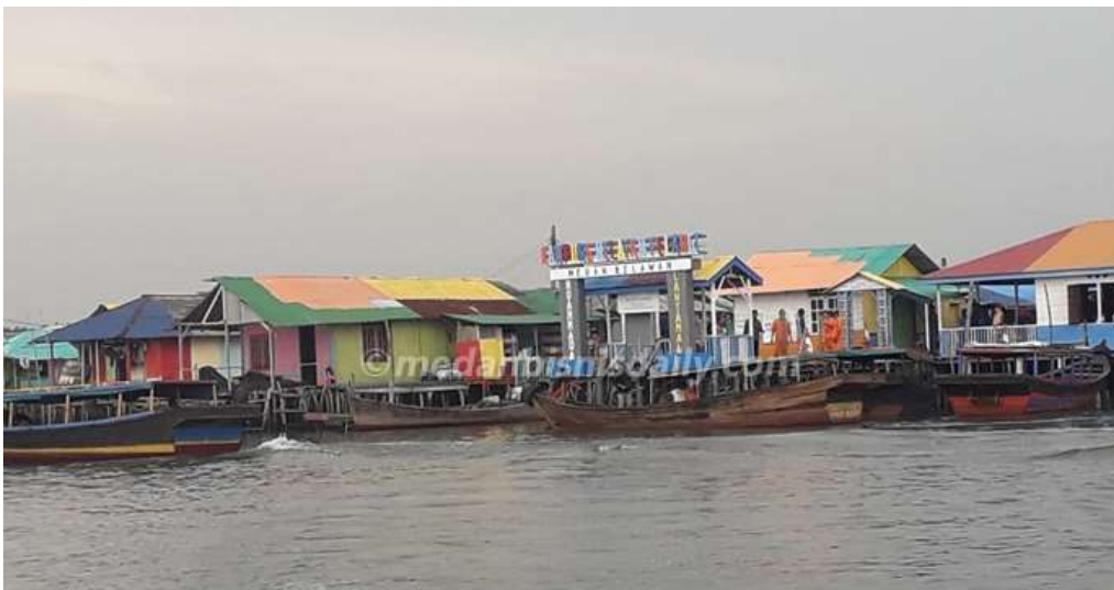
Figure 4.1 Condition of Settlement in Seberang Fisherman's Village
