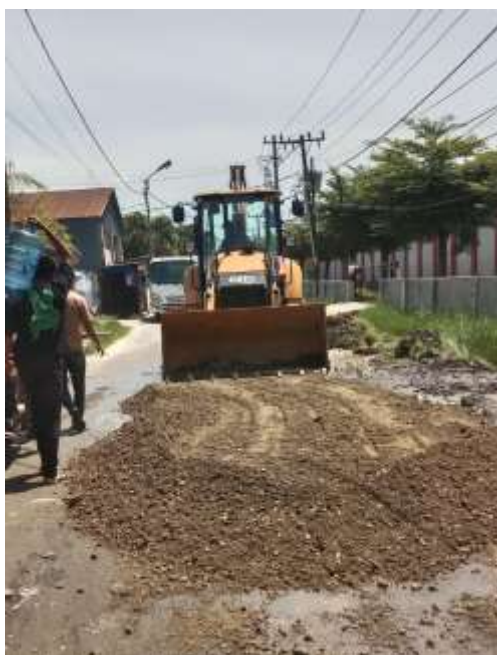
Figure 4.8 Routine maintenance of city roads
