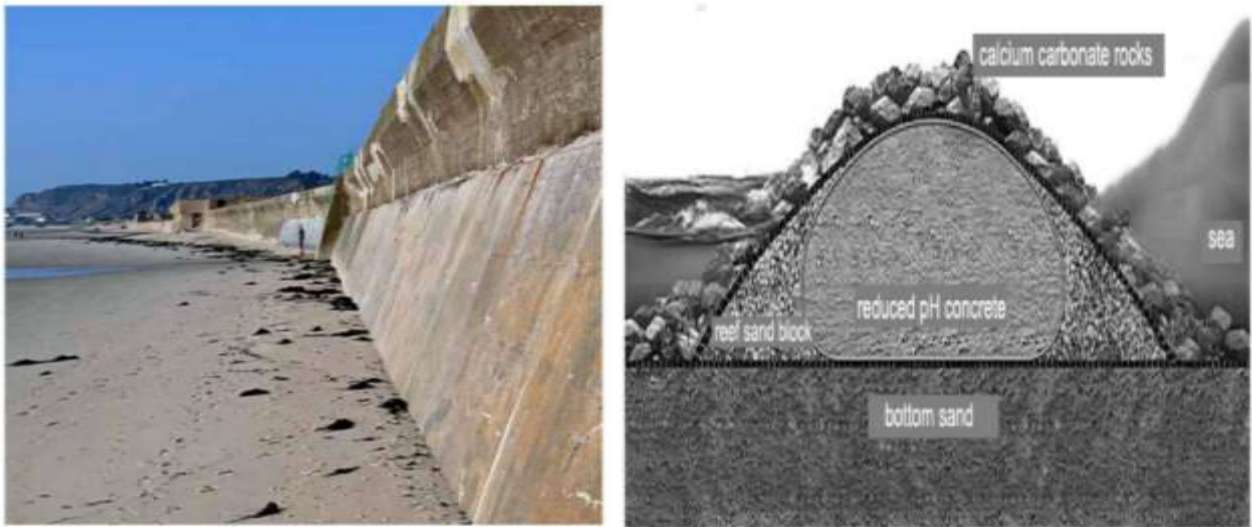
Figure 2.1 1of hard engineering of coastal barriers (seawalls)
