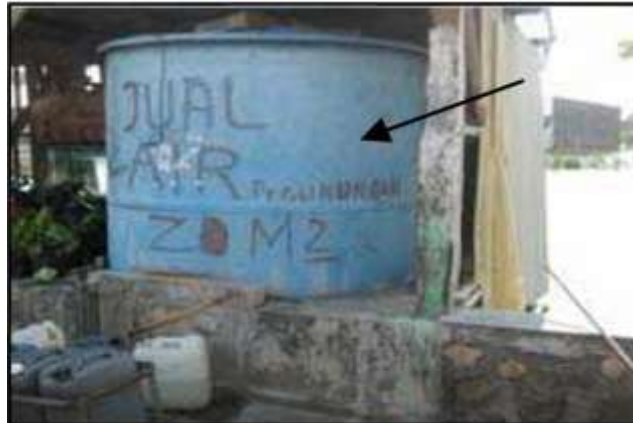
Figure 2.6 Clean water storage tank
