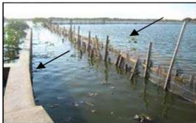
Figure 2.7 Concrete embankment and net in pond
