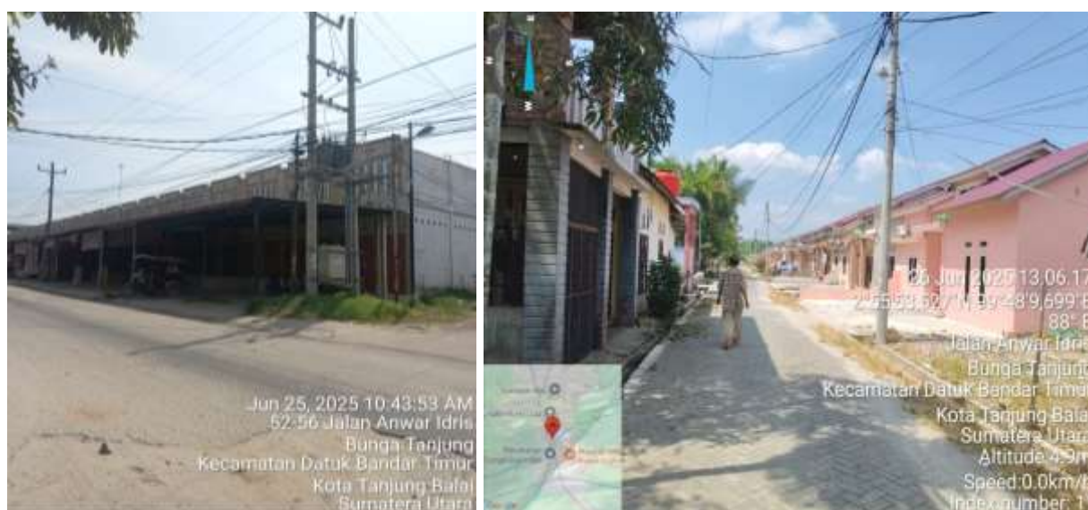
Figure 4.3 Housing in Datuk Badar Timur District
