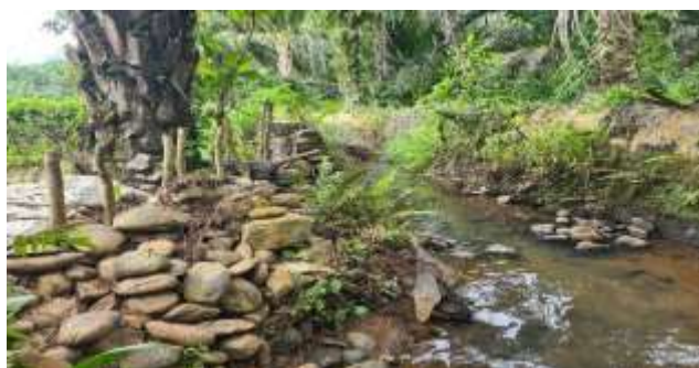
Figure 4.2. Damage to the Primary Channel Causing Reduced Water Distribution
