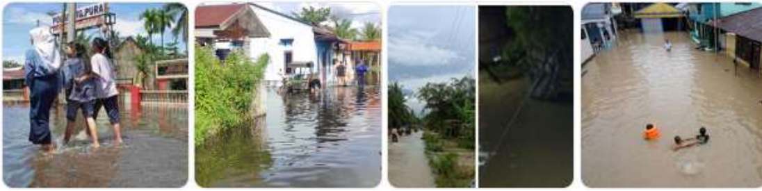
Figure 4.2 Overview of the Existing Condition of the Sanitation System in Tanjung Pura District, Langkat Regency
